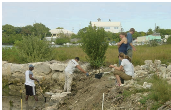
Figure 6. Building revetment and planting native red mangrove.
