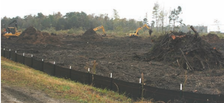
Figure 9. The bulldozed site
